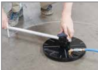
Set up vacuum base and mark cut with soap stone by rotating pivot bar
